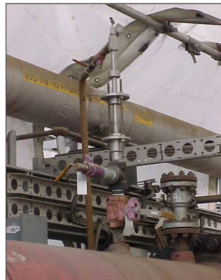
Figure 4: High Pressure Sparger
