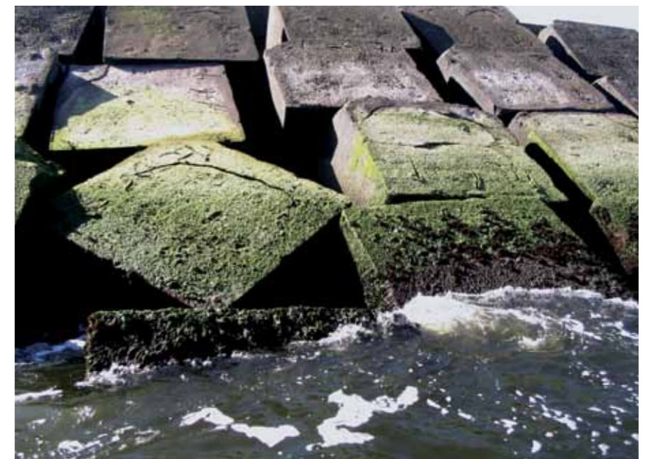
Photo above: armour stone with coarse grading. Photo below: armour stone with heavy grading.
